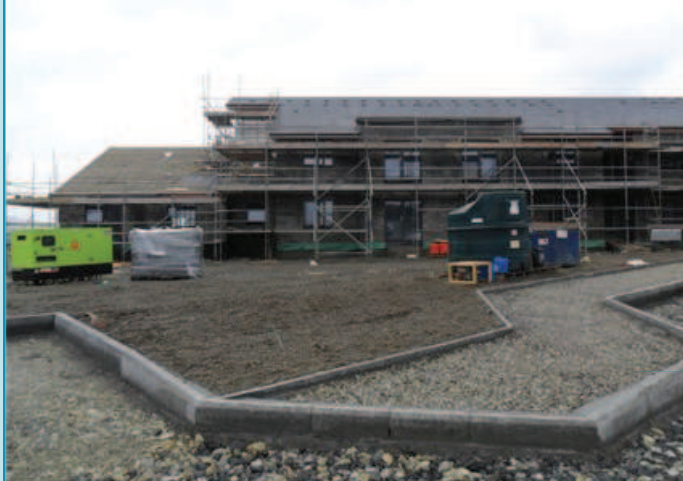
Mull Progressive Care Centre under construction
